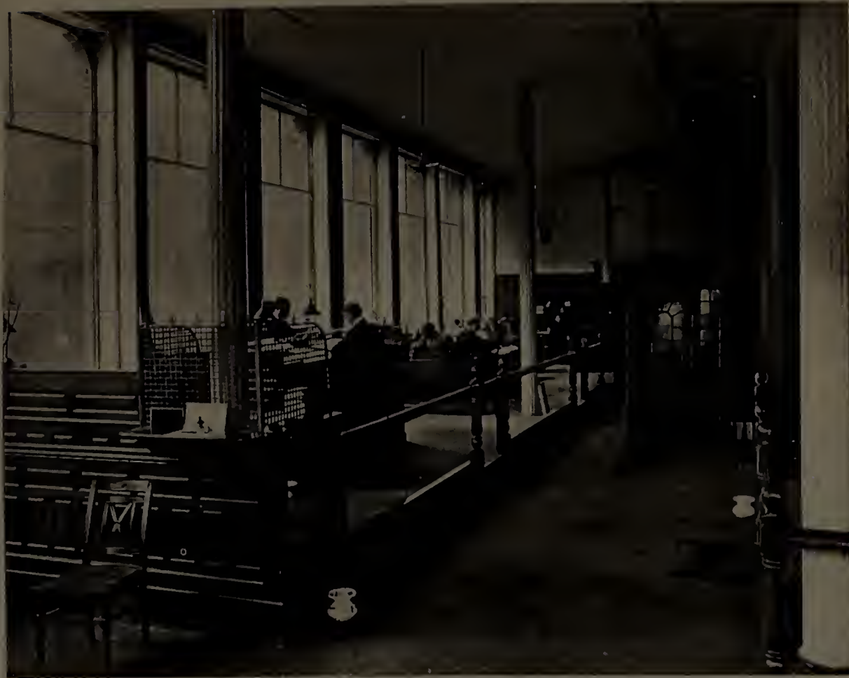
OFFICES UNITED STATES RUBBER COMPANY, corner Chauncy and Bedford Streets.
